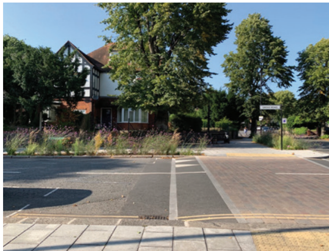
Figure 3.4 The photos show two of the raingardens built on College Road, designed to capture rain water from the surrounding roads and reduce peak flows into the sewer network.
